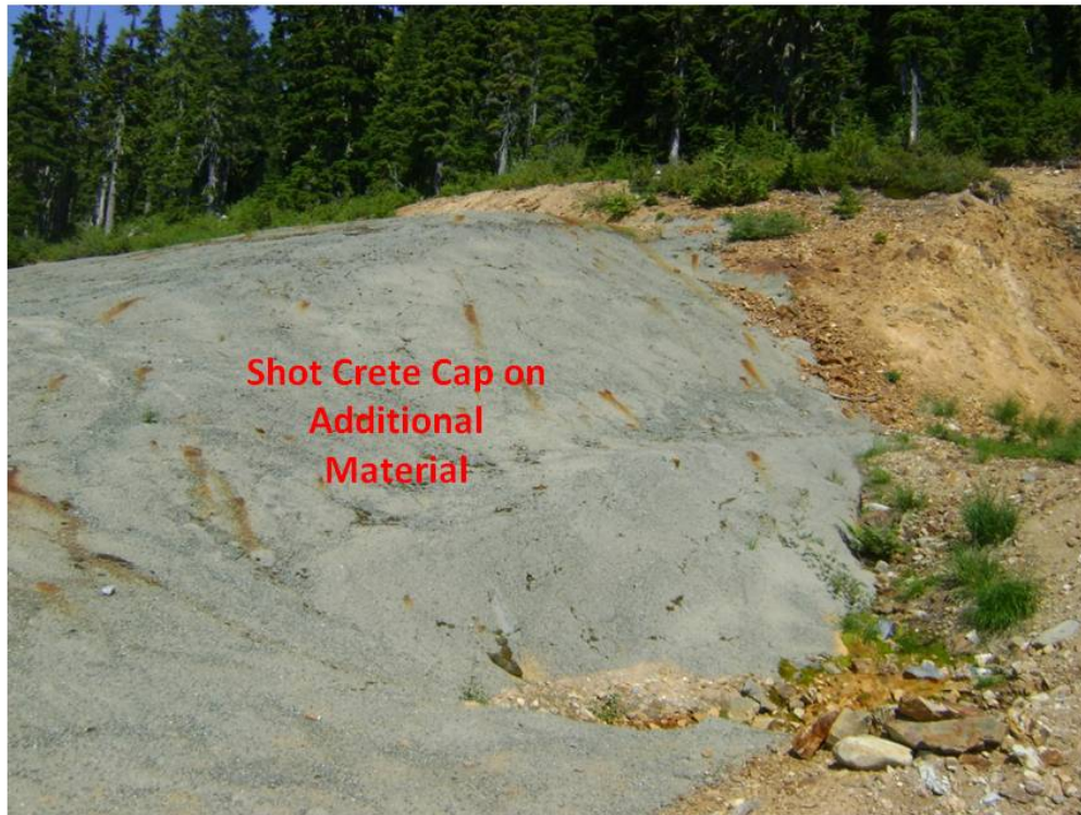
Fig 7 – Bulk Sample covered by shotcrete
